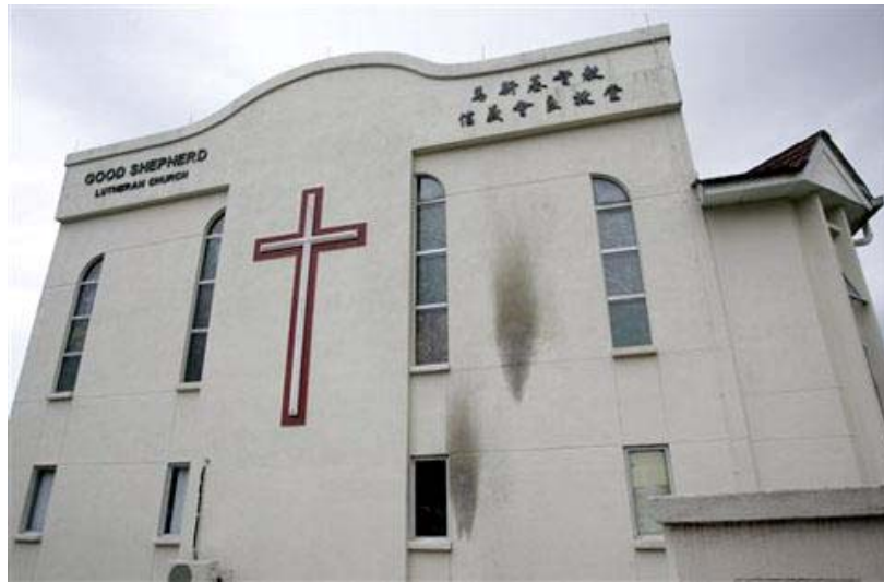
Damage to the exterior of the Good Shepherd Lutheran Church in Petaling Jaya, near Kuala Lumpur (Photo credit: VOA News 7 )
